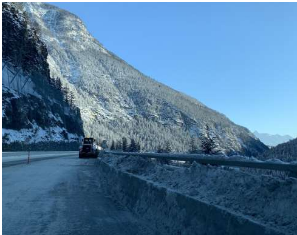
Figure 2: Loader cleaning snow from barrier – January 2024
