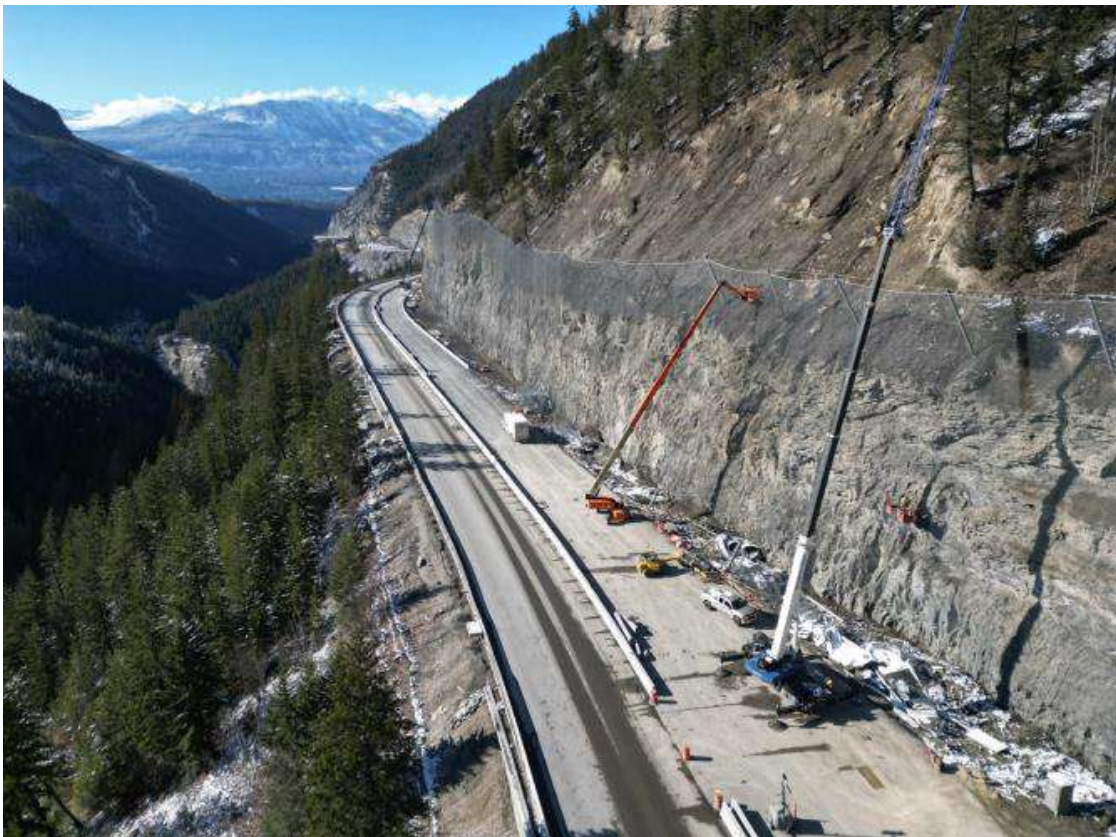
Figure 6: Cut 4 – Rock attenuator installation ongoing
