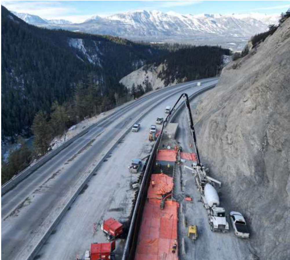
Figure 3: Sheep Bridge – Avalanche wall installation ongoing
