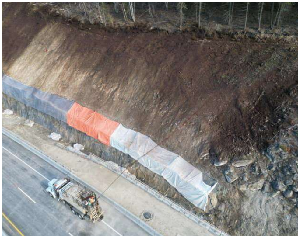
Figure 2: Bison Upslope Wall – Hydroseeding ongoing
