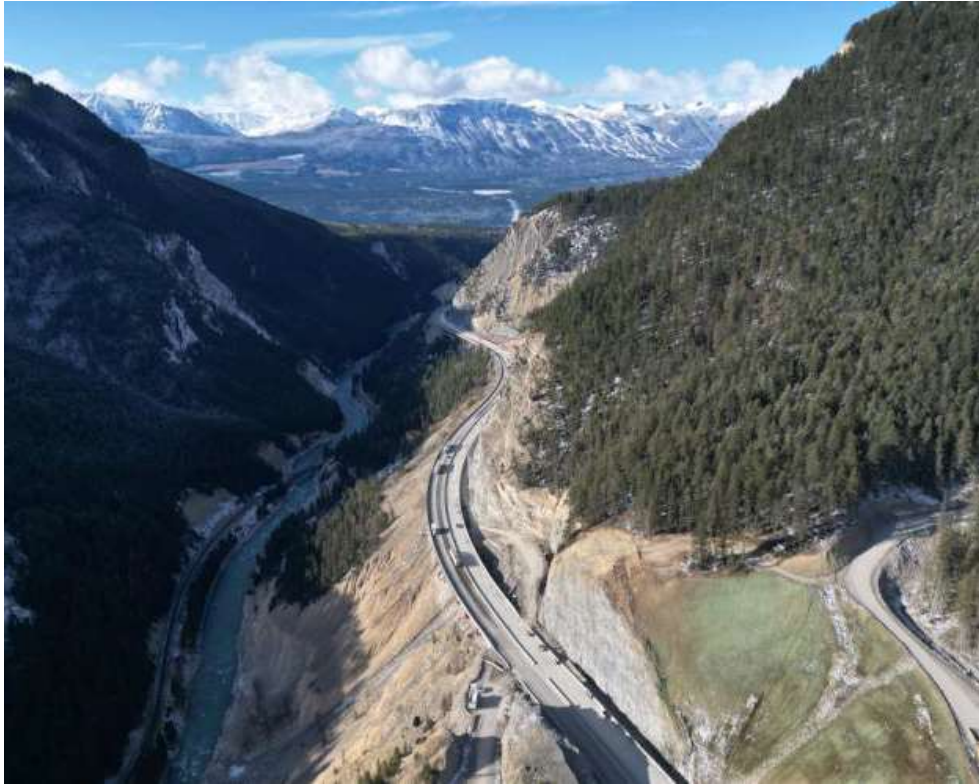
Figure 1: Cut 3 – Looking east
