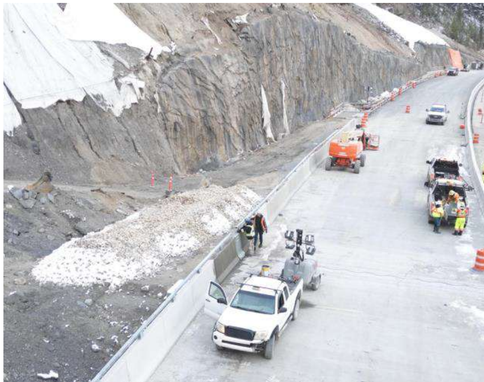
Figure 4: Hedgehog Viaduct – Parapet wall finishing ongoing
