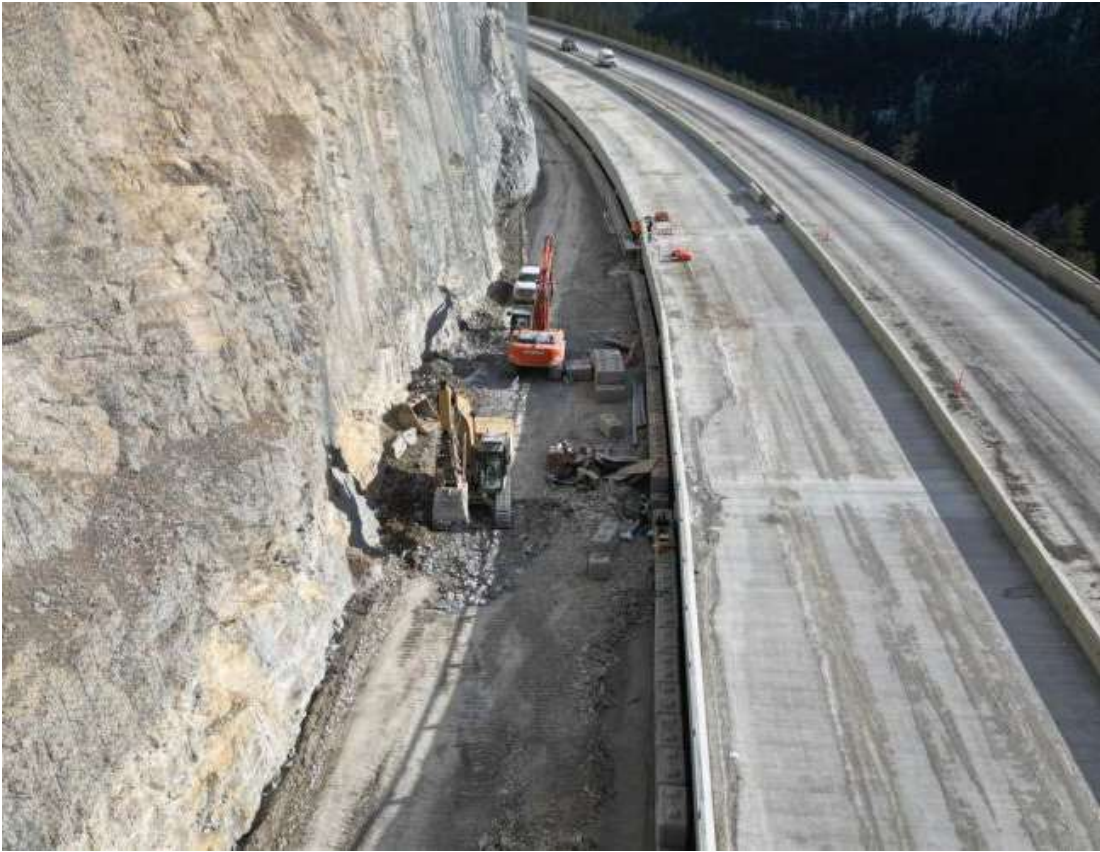
Figure 5: Lynx Viaduct– Avalanche wall installation ongoing
