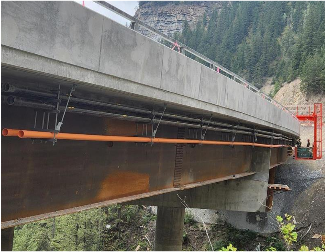
Figure 5: Blackwall Bridge – Utility duct installation under bridge ongoing – August 22, 2023
