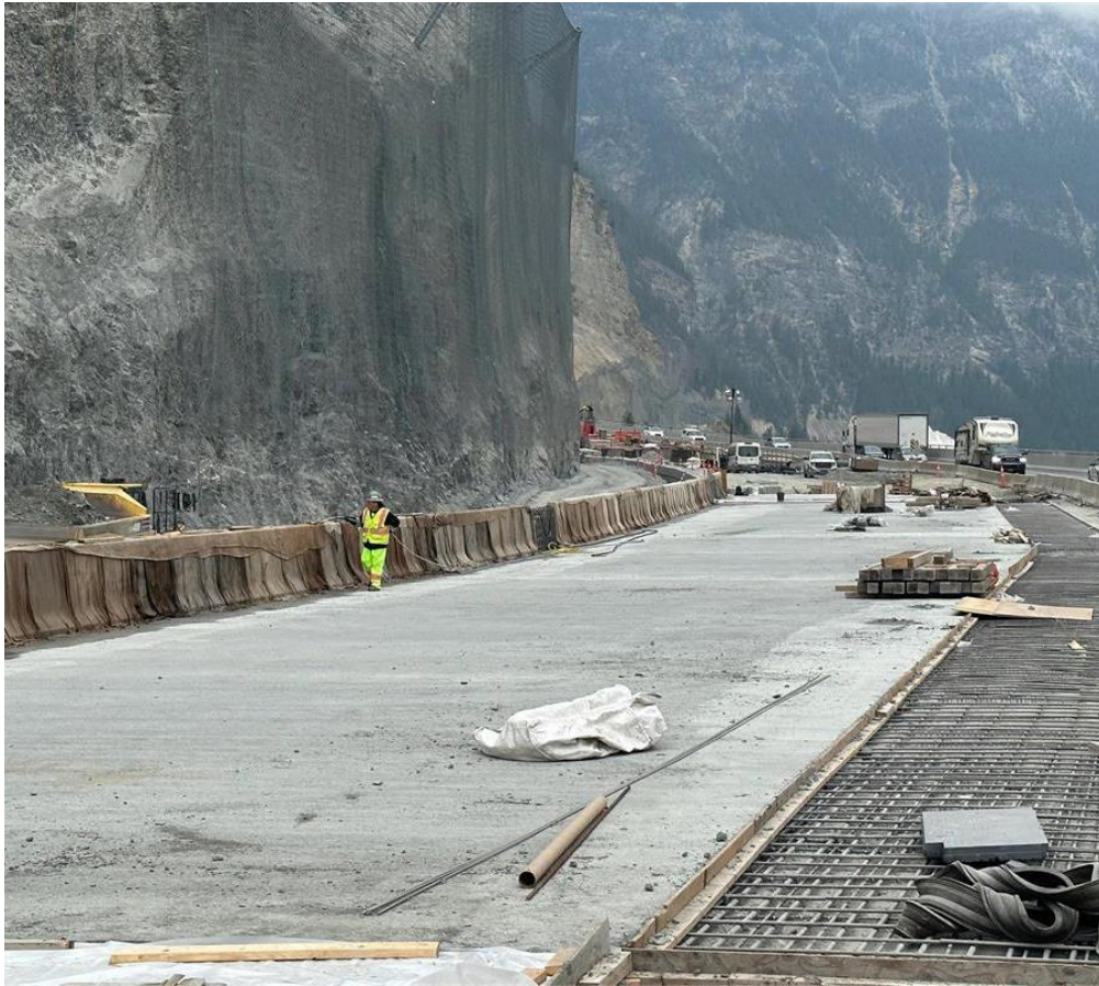
Figure 3: Sheep Bridge – Deck and parapet construction ongoing – August 31, 2023
