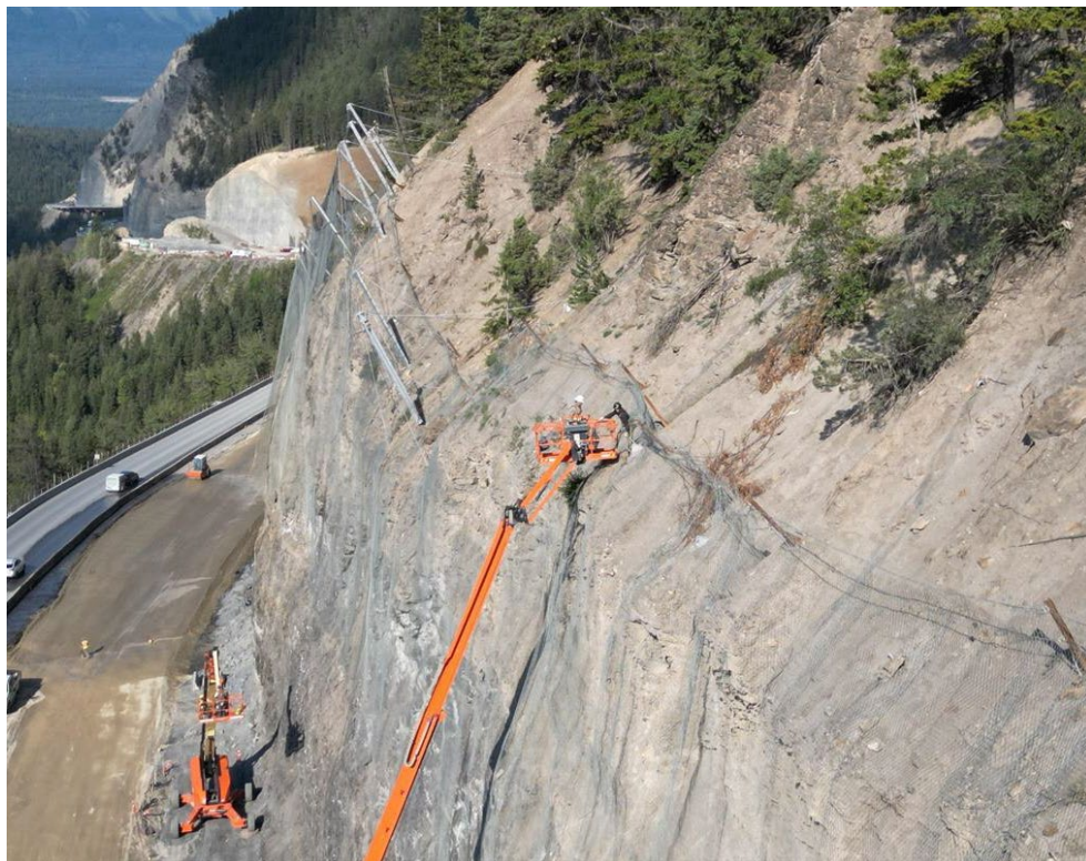
Figure 2: Cut 4 – Crew installing rock attenuator fencing – July 28, 2023
