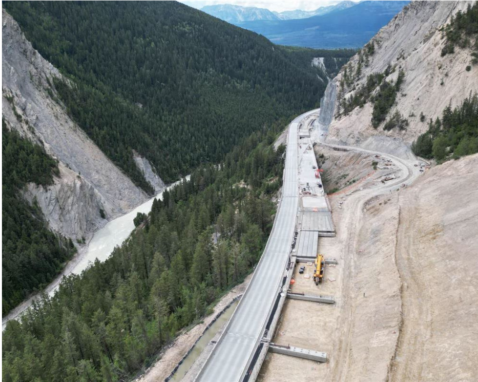
Figure 1: Lynx Viaduct – Stringer installation ongoing – July 28, 2023
