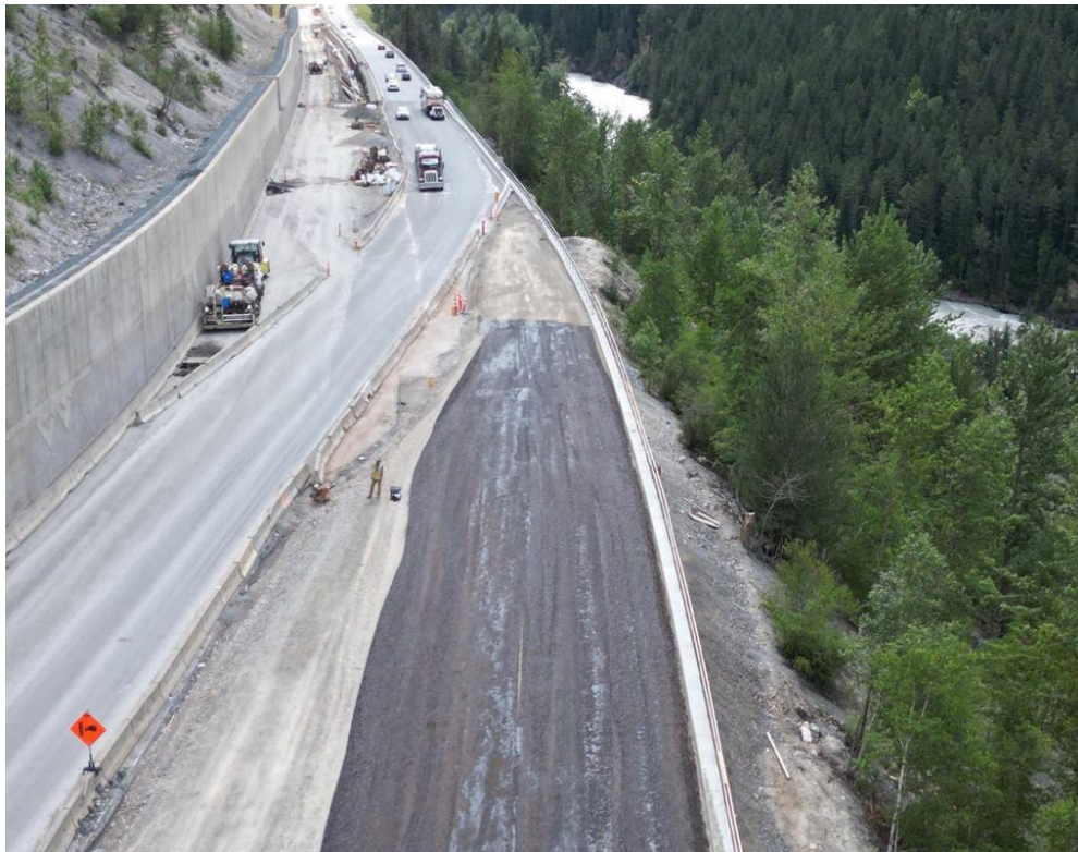
Figure 4: Caribou Wall – Preparing asphalt surface to merge into eastbound lanes – July 28, 2023
