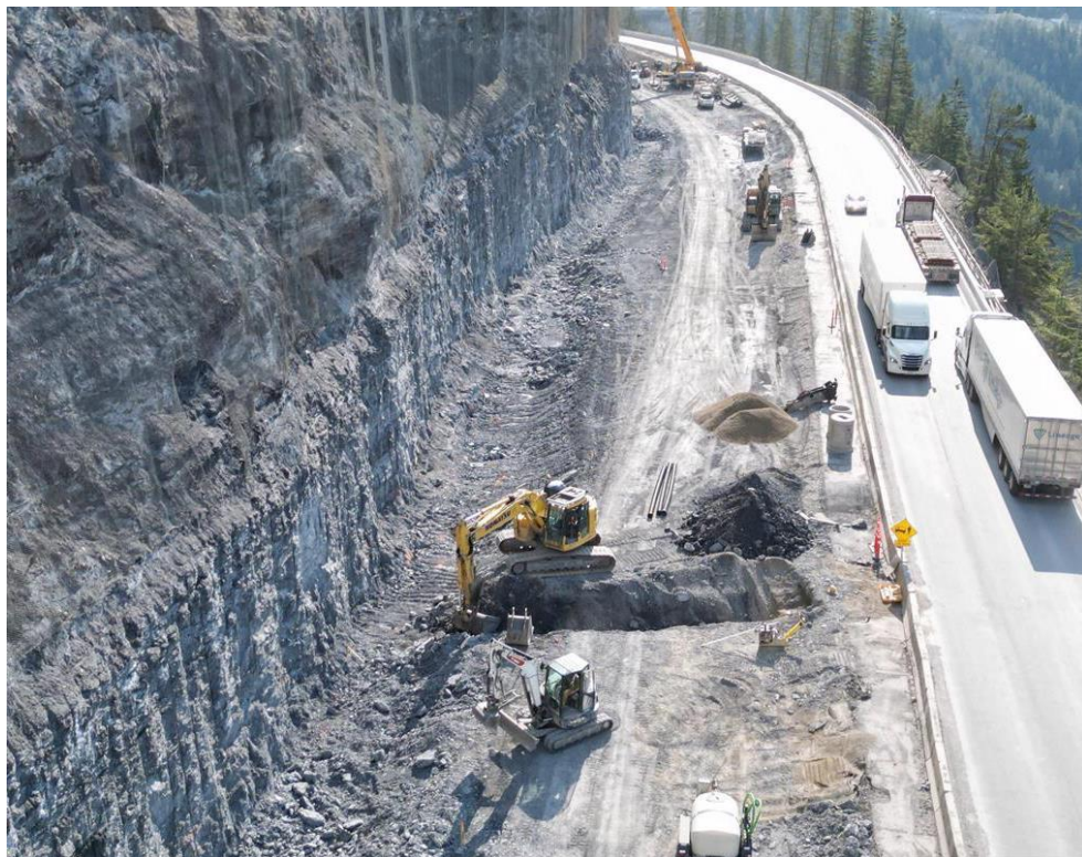
Figure 2: Cut 4 – Crew installing storm water drainage – June 27, 2023
