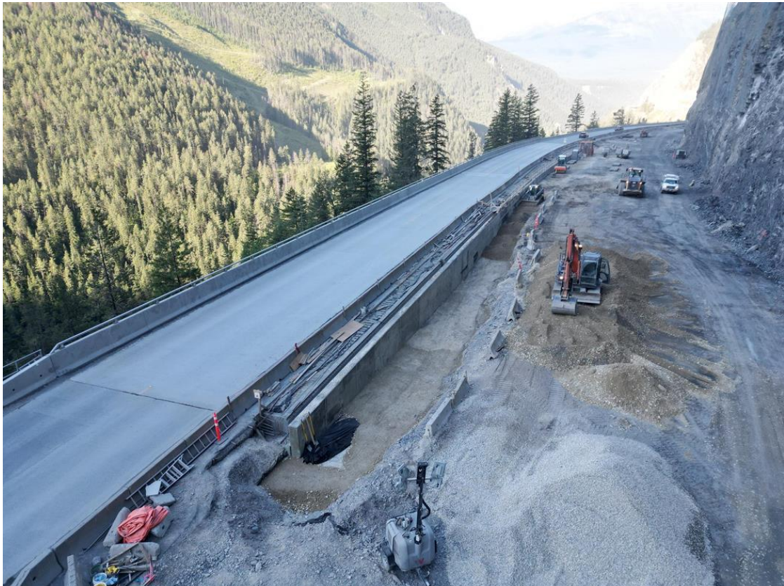
Figure 6: Wolf Viaduct – Civil crew back-filling median wall – June 30, 2023
