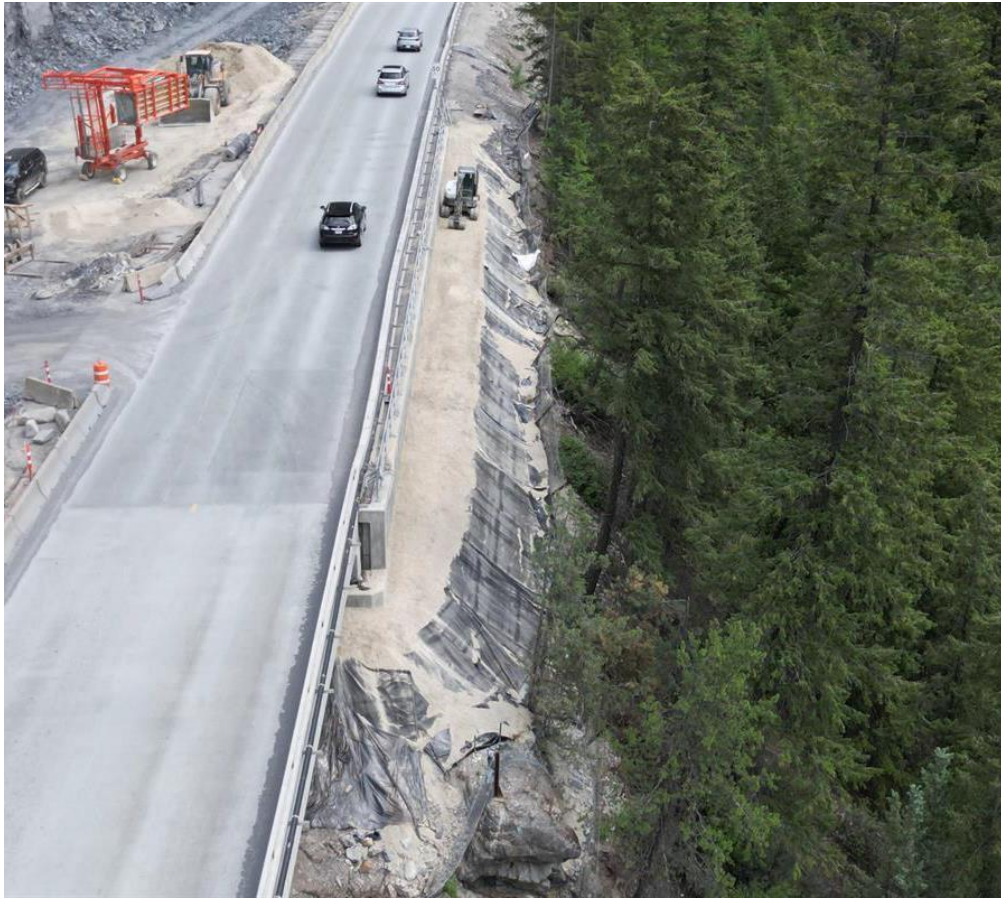
Figure 3: Grizzly Wall 3 – Geo-membrane backfill operation ongoing – June 29, 2023
