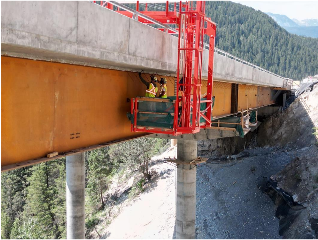
Figure 5: Bighorn Bridge – Concrete finishing the underside of the bridge – June 28, 2023
