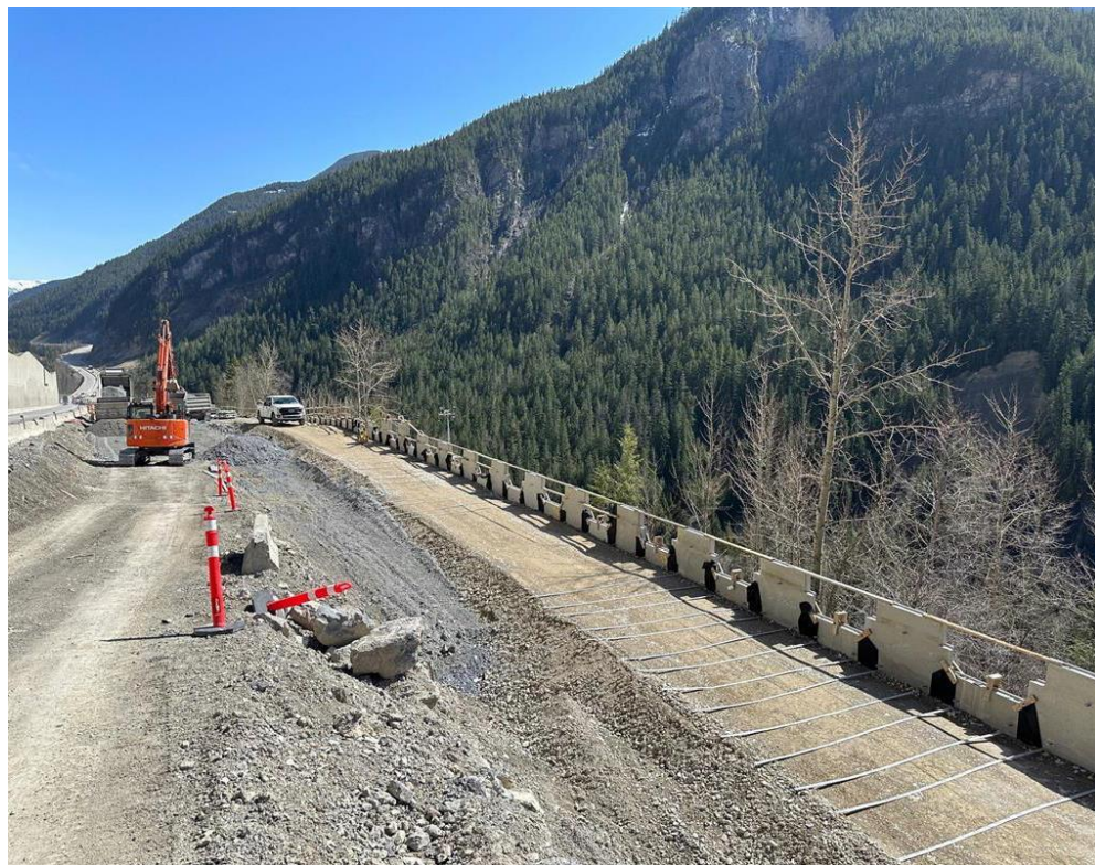
Figure 4: Caribou Wall – MSE Wall strap installation and backfilling ongoing – April 28, 2023
