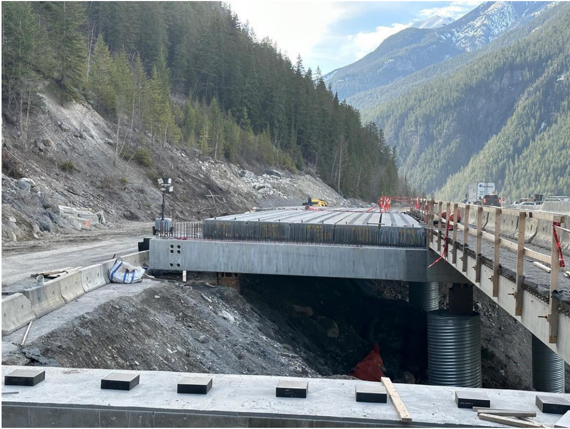
Figure 5: Marmot Viaduct – Precast stringer installation ongoing – April 28, 2023
