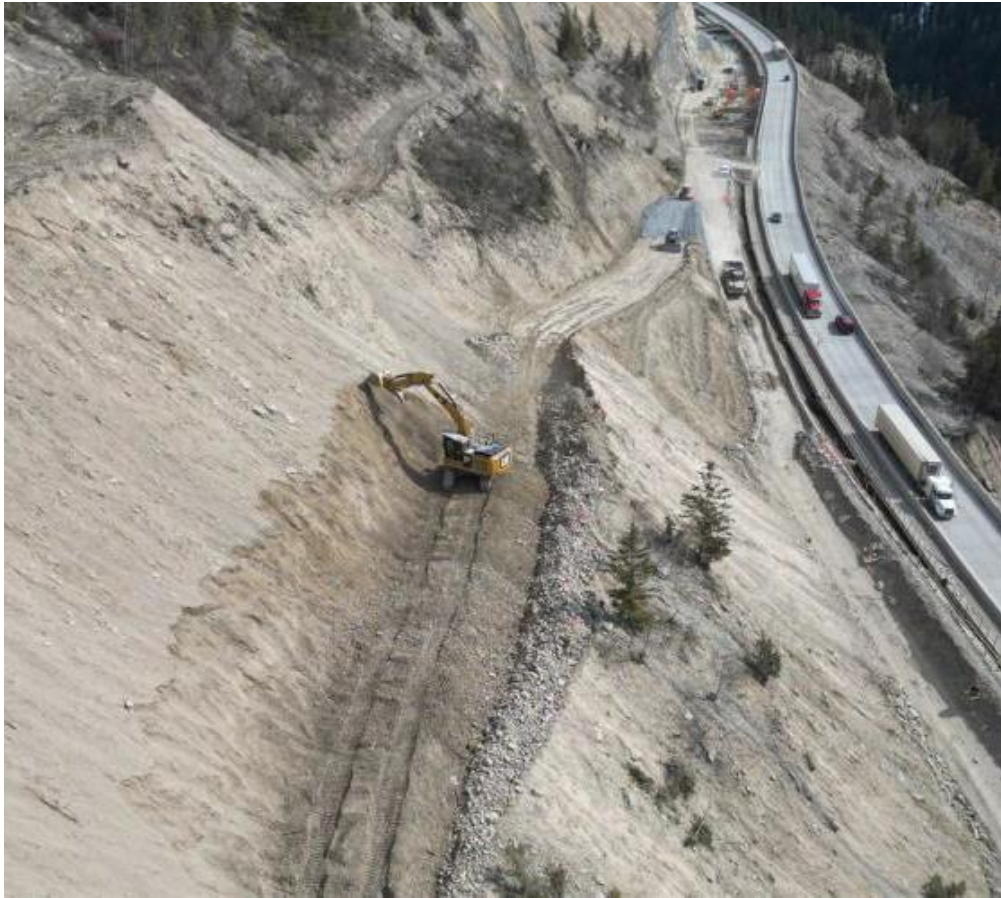
Figure 3: Pronghorn Upslope – Crews continue to widen the middle bench – March 29, 2023
