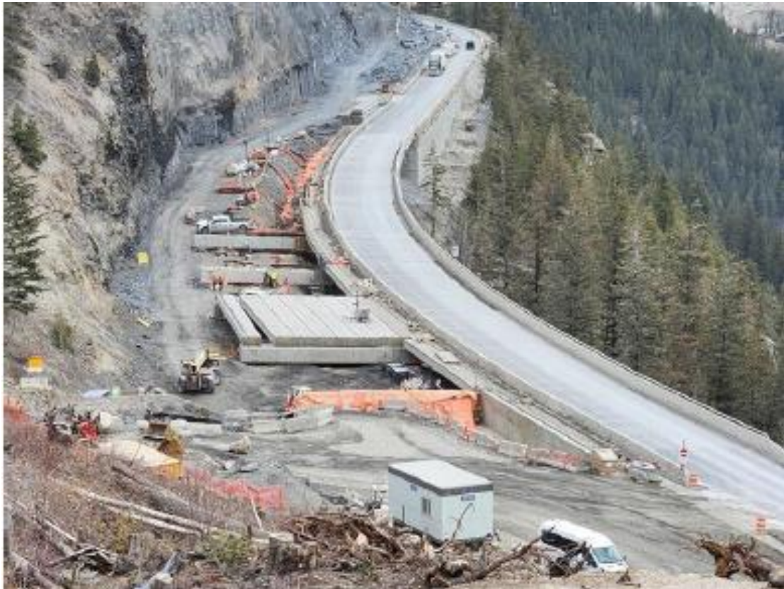
Figure 6: Elk Viaduct – Pier 2 and 3 works ongoing – March 31, 2023
