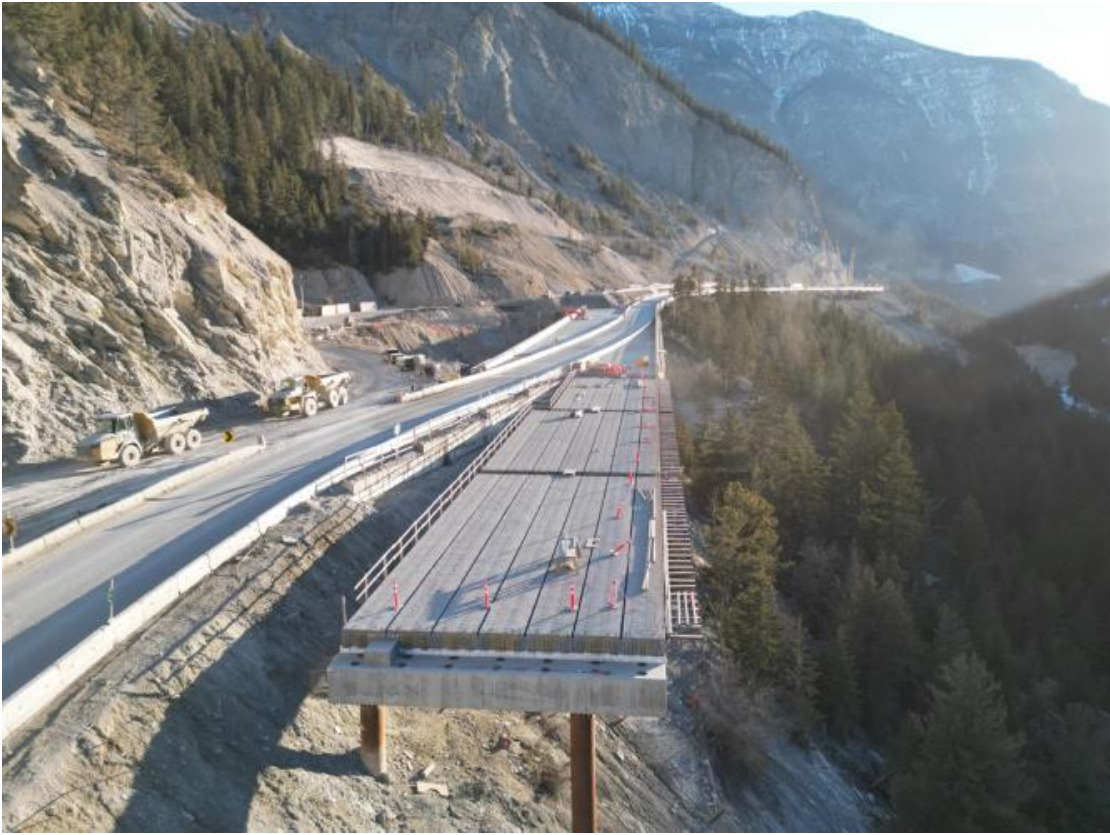
Figure 5: Bighorn Viaduct – View looking east – March 28, 2023
