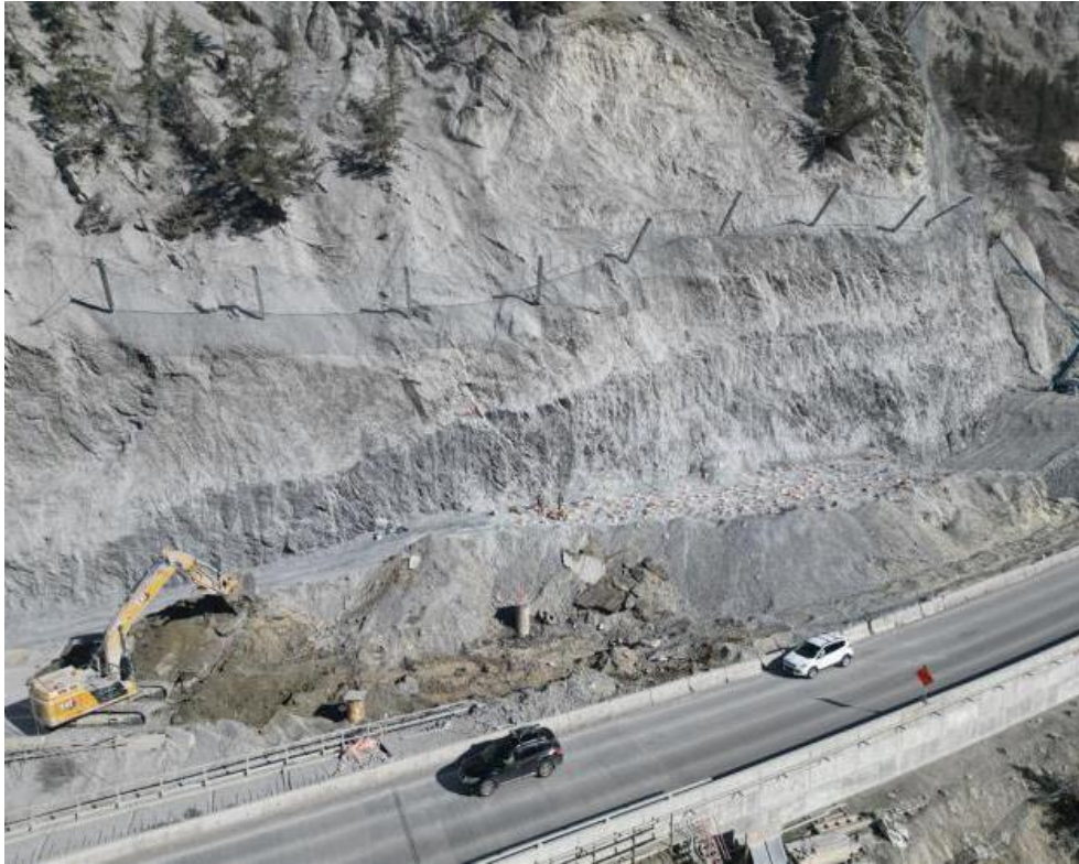
Figure 1: Cut 1 – Excavator pioneering to the east abutment piles – March 30, 2023
