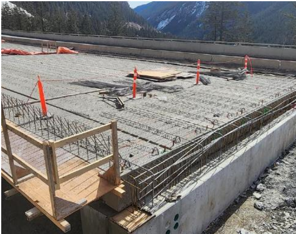
Figure 4: Grizzly Viaduct – Rebar installation on west end of deck – March 29, 2023
