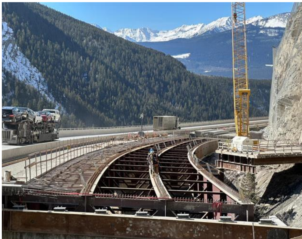
Figure 2: Frenchman's Bridge – Survey in progress – March 30, 2023
