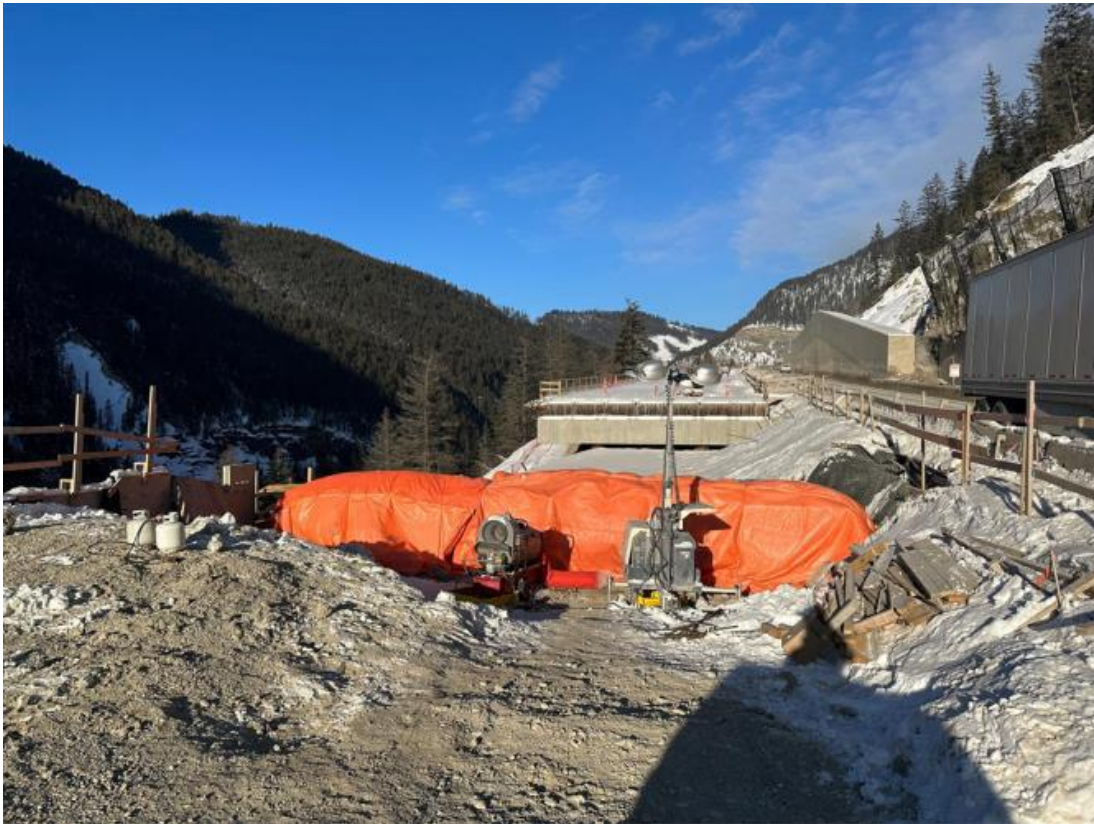
Figure 6: Caribou Viaduct- Installation of east and west abutments continue – February 24, 2023
