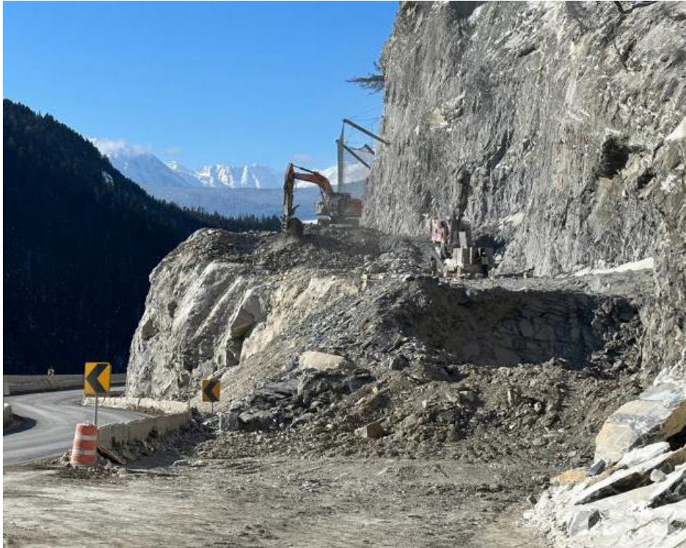
Figure 1: Cut 1 – Blasting and excavation ongoing – February 24, 2023
