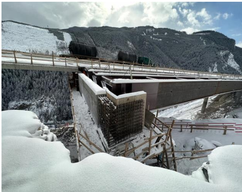
Figure 2: Frenchman's Bridge – Rebar installation for westbound transition pier – February 27, 2023
