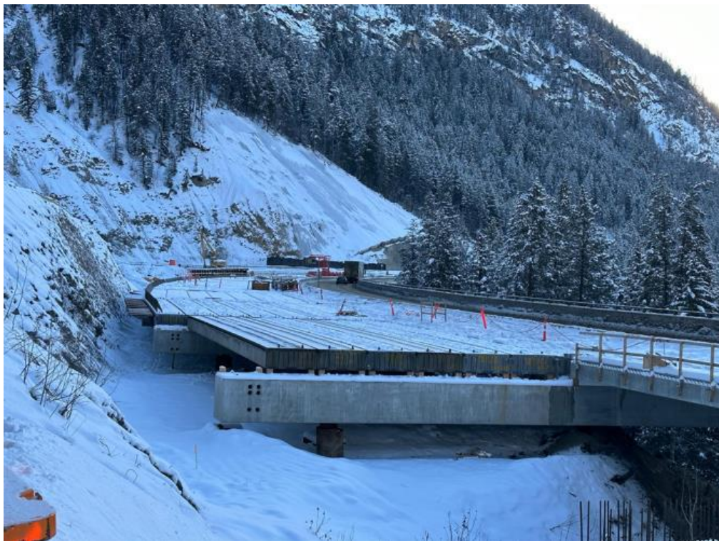
Figure 4: Grizzly Viaduct – Pre-cast stringers installation ongoing – February 28, 2023
