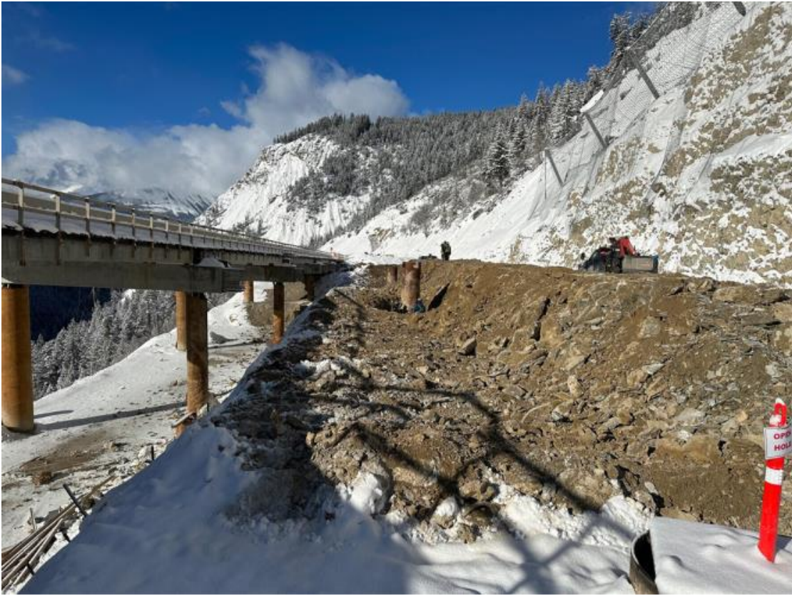
Figure 5: Lynx Viaduct –Pile installation ongoing – February 27, 2023
