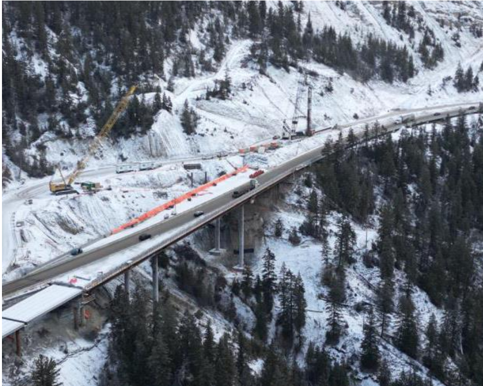
Figure 1: Bighorn Bridge – Traffic heading through site on the new alignment – November 26, 2022
