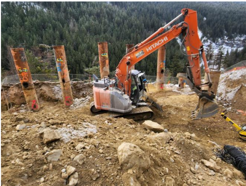
Figure 4: Caribou Viaduct - Ground preparation for eastbound abutment – November 26, 2022
