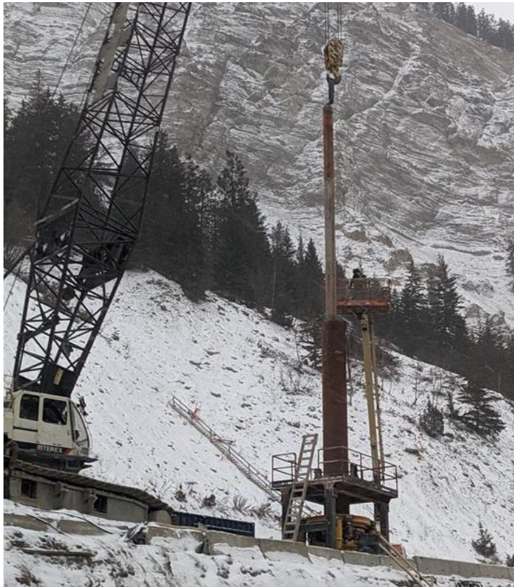
Figure 6: Lynx Viaduct – Crews installing piles – November 30, 2022
