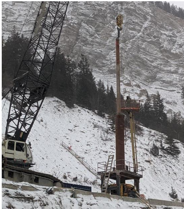
Figure 6: Lynx Viaduct – Crews installing piles – November 30, 2022
