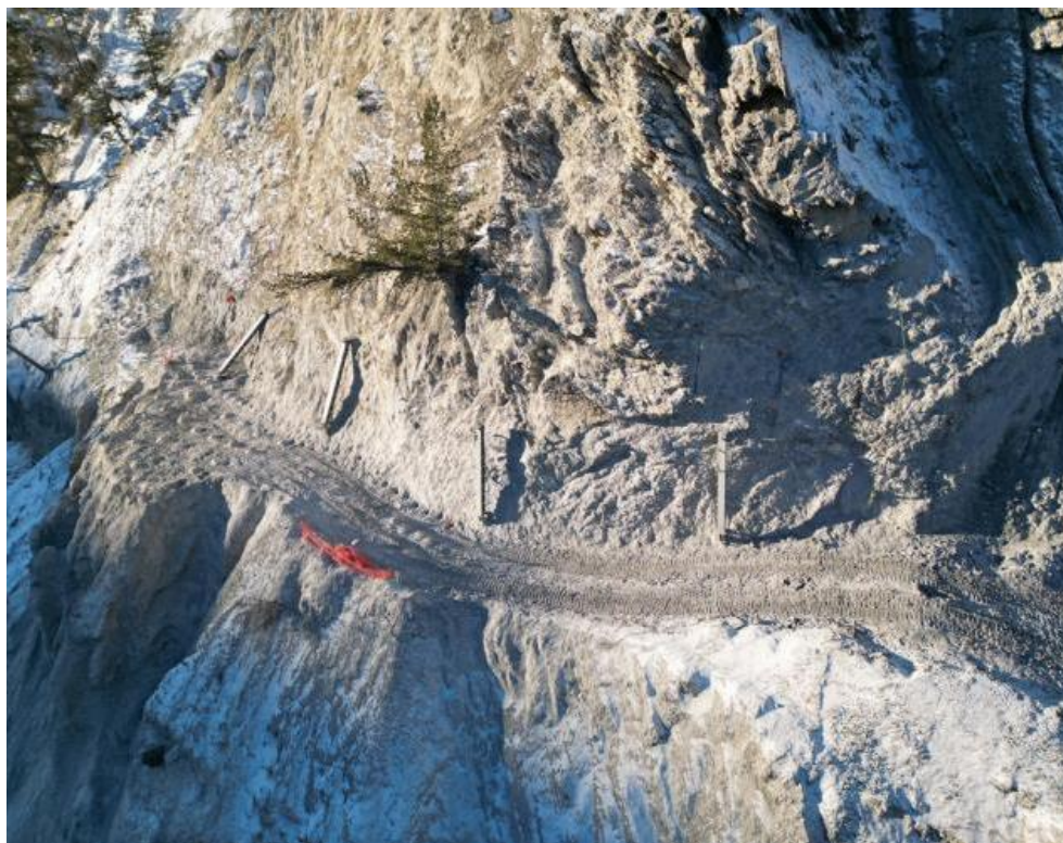
Figure 2: Cut 1 – Crews installing attenuator posts – November 28, 2022
