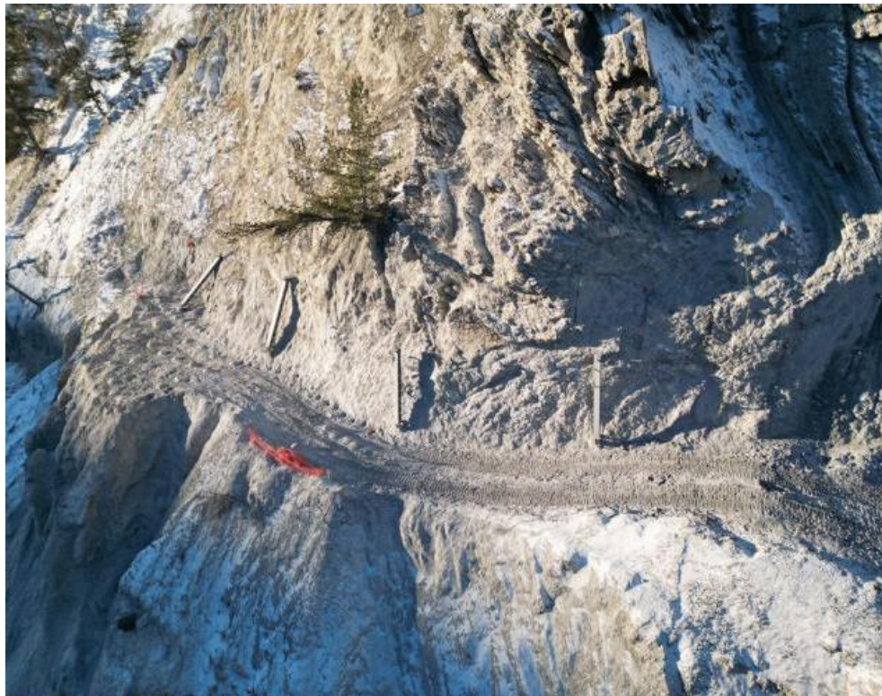
Figure 2: Cut 1 – Crews installing attenuator posts – November 28, 2022
