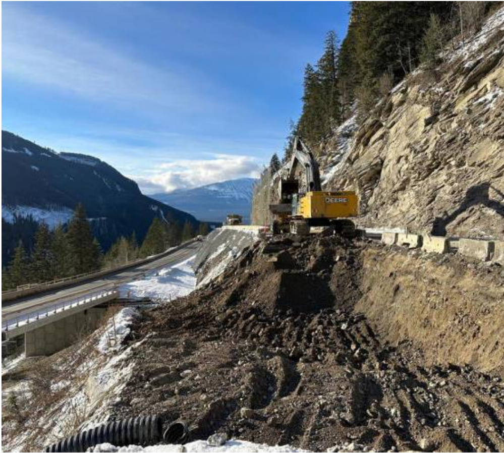
Figure 3: Cut 4 – Excavation of old highway at east end – November 28, 2022
