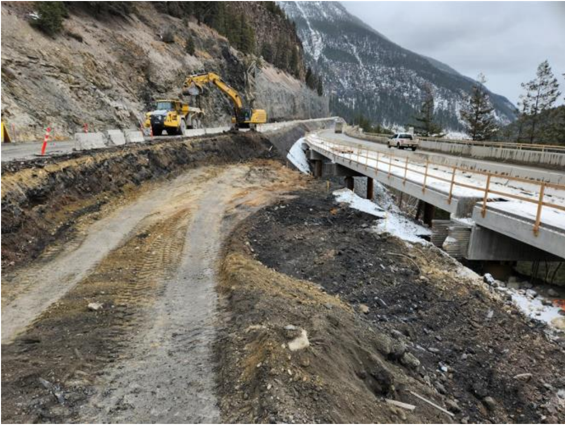
Figure 5: Elk Viaduct - Excavation of future westbound lanes of the Viaduct – November 25, 2022
