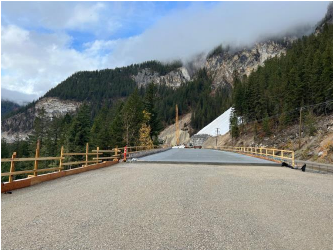
Figure 6: Marmot Viaduct - Western approach – October 28, 2022
