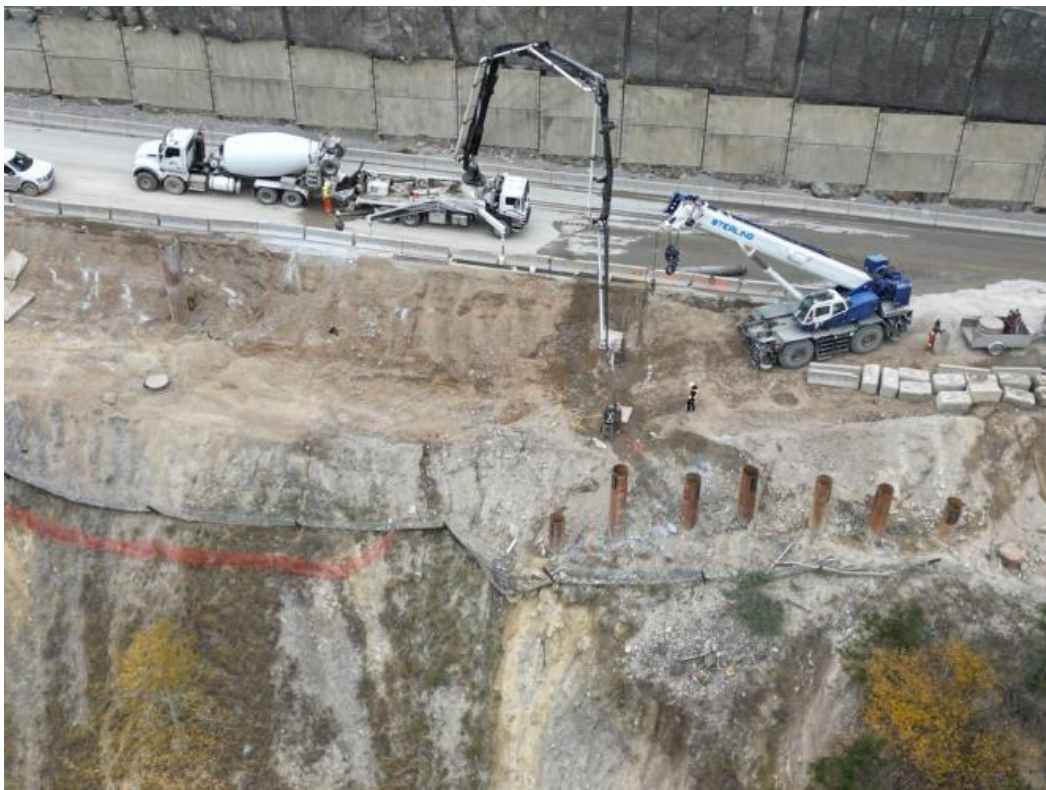
Figure 4: Caribou Viaduct -Crews pouring concrete into piles – October 27, 2022
