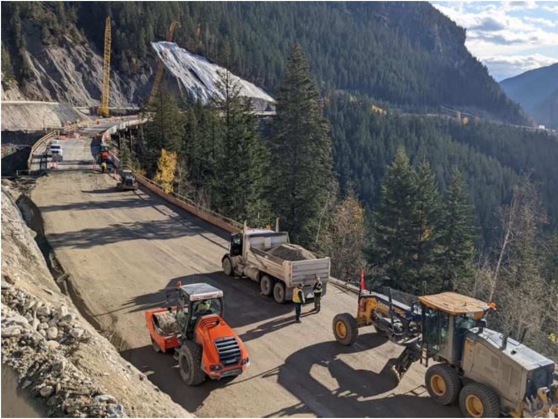
Figure 5: Grizzly Wall 4 - Crews installing, grading and compacting road base – October 29, 2022
