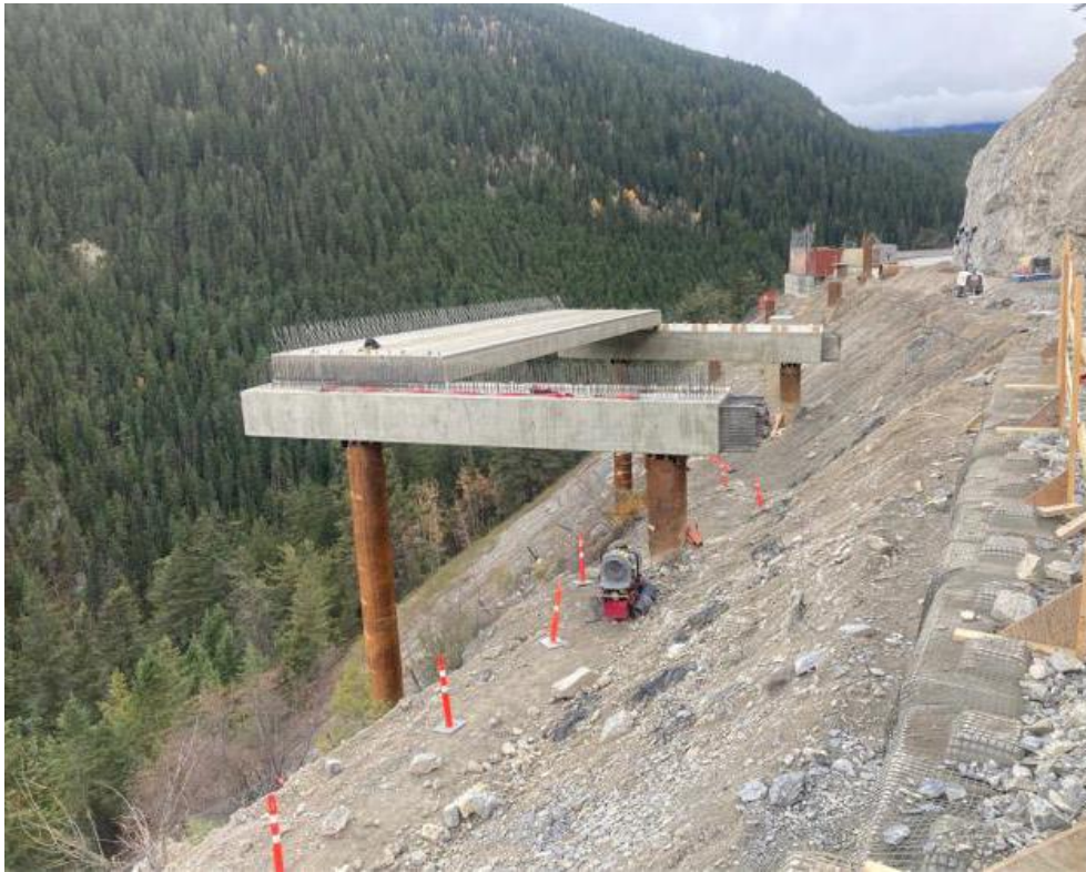
Figure 1: Bighorn Viaduct – Pre-cast stringer installation – October 31, 2022
