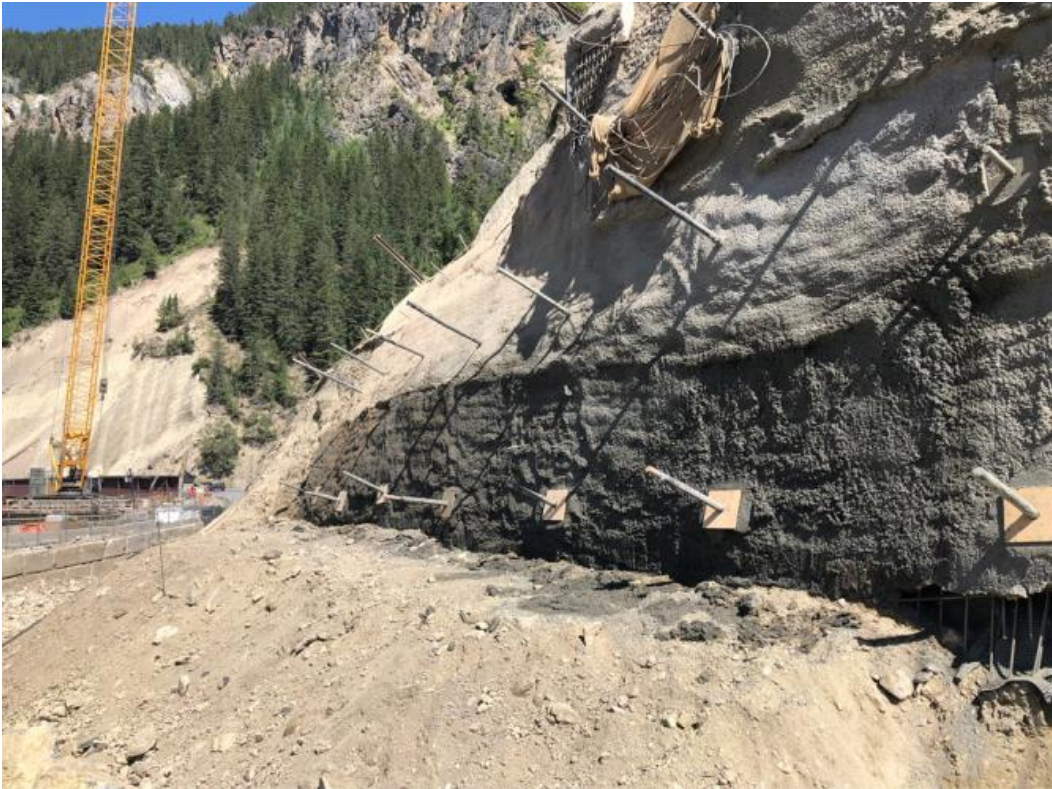
Figure 4: Bison Upslope Wall – Shotcrete and soil anchor installation ongoing – July 26, 2022
