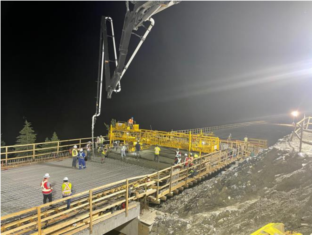
Figure 3: Lynx Viaduct – Start of deck pour – July 29, 2022
