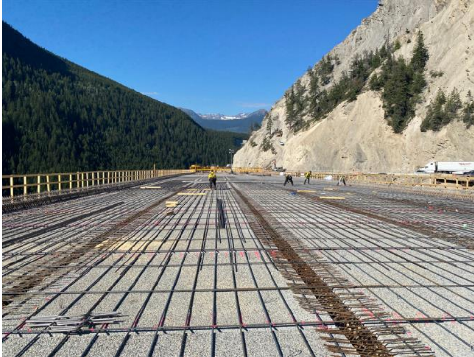
Figure 1: Bighorn Bridge – Harris rebar installation ongoing – July 28, 2022
