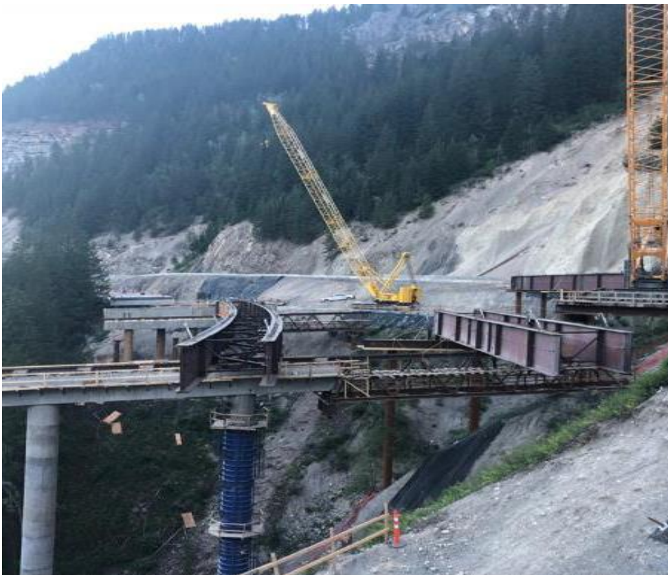
Figure 2: Blackwall Bridge – Girder installation in progress – July 27, 2022
