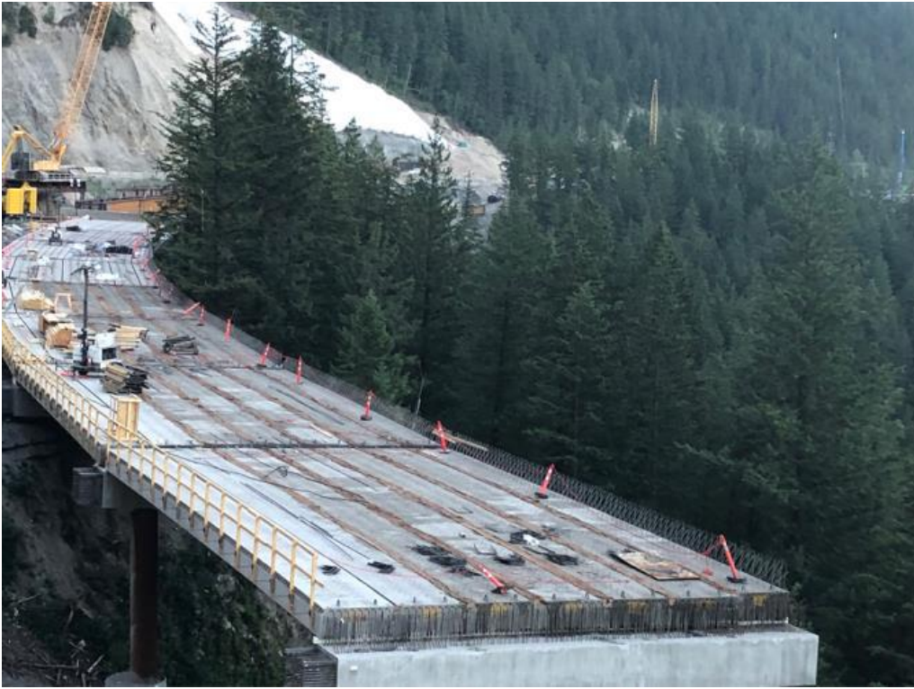
Figure 5: Grizzly Viaduct – Stringer installation in progress – July 26, 2022
