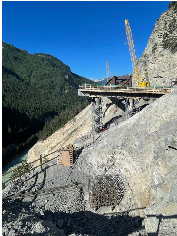
Figure 6: Frenchman's Viaduct – Reinforcement pad installation ongoing – July 26, 2022
