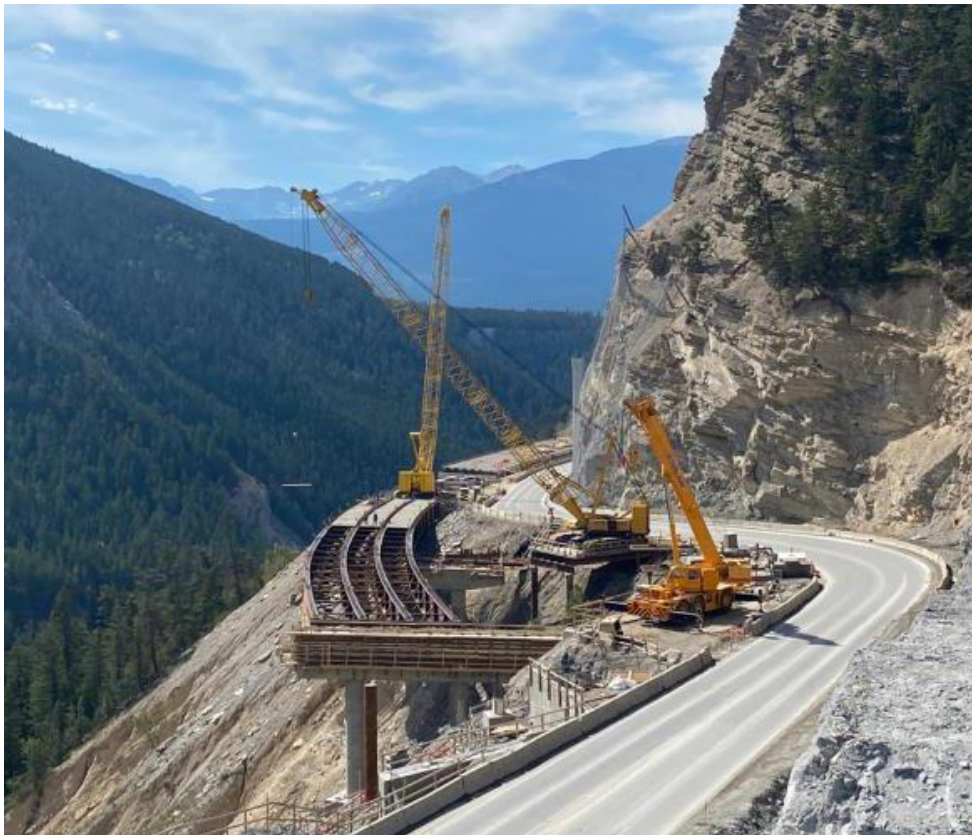
Figure 2: Frenchman's Bridge – Deck installation in progress – August 30, 2022
