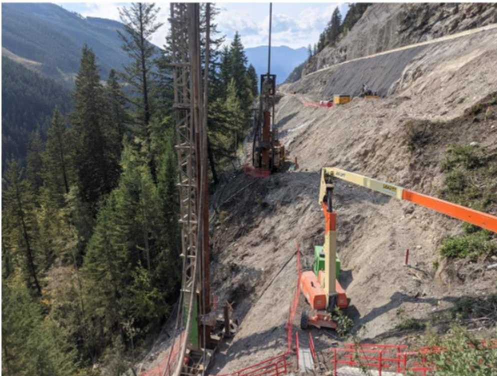
FIGURE 2: GRIZZLY 4 – CDI CREWS INSTALLING TRESTLE PILES – SEPT 10, 2021
