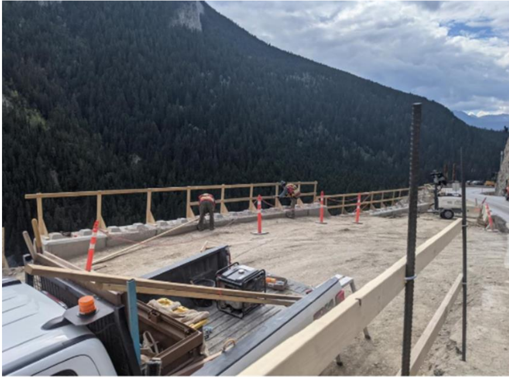
FIGURE 3: BIGHORN WALL – KHCC CREWS CONSTRUCTING SAFETY RAILINGS – SEPT 11, 2021
