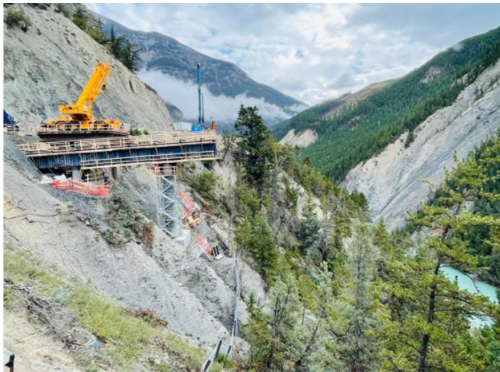
FIGURE 4: SHEEP'S BRIDGE- CONCRETE PIER CAP CONSTRUCTION AT PIER 2 – SEPT 15, 2021
