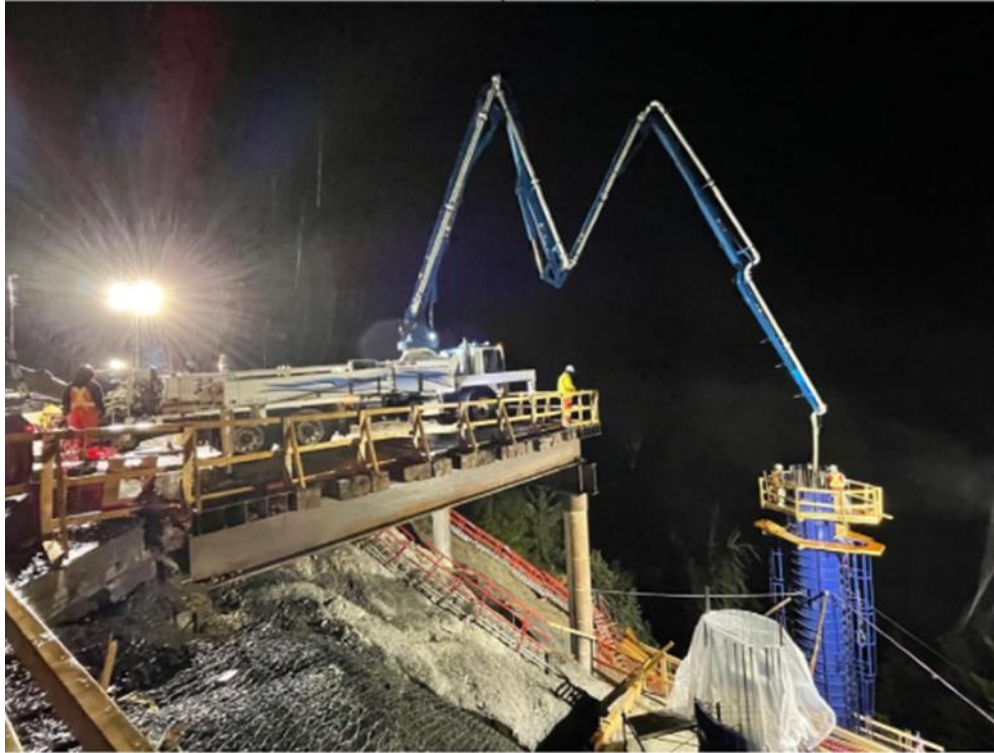
FIGURE 1: SHEEP'S BRIDGE – POURING COLUMNS AT PIER 2 SOUTH AND NORTH – SEPT 1, 2021
