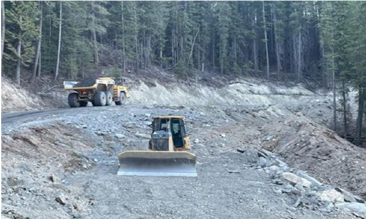
Figure 4: Ongoing embankment construction and forest service road maintenance
