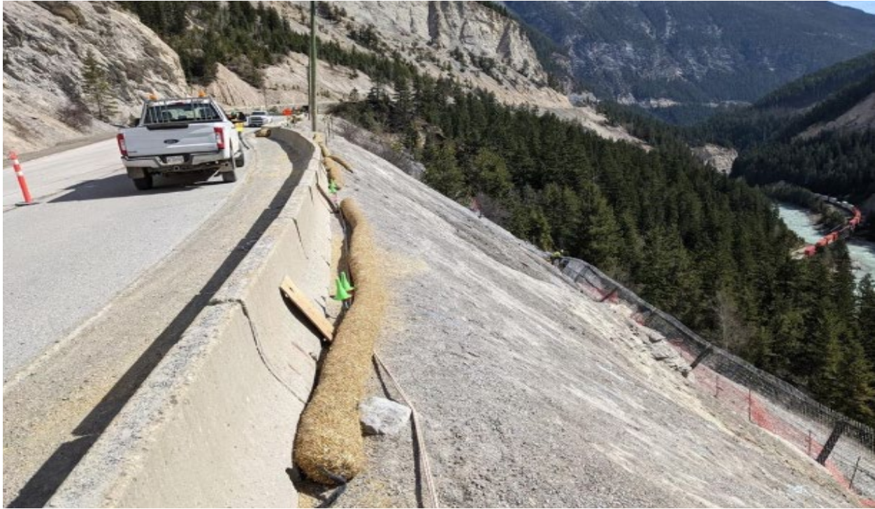
Figure 3: BCIB crews installing sediment control measures at Bighorn
