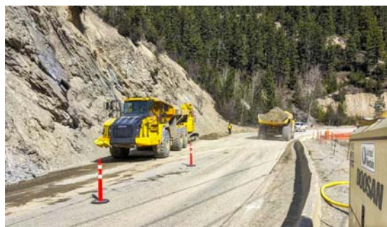
Excavated materials being hauled away.
