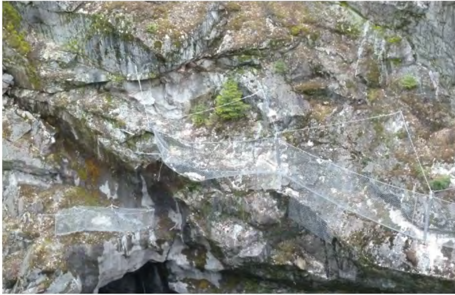
GBE-500A rockfall barrier protecting the tunnel entrance
