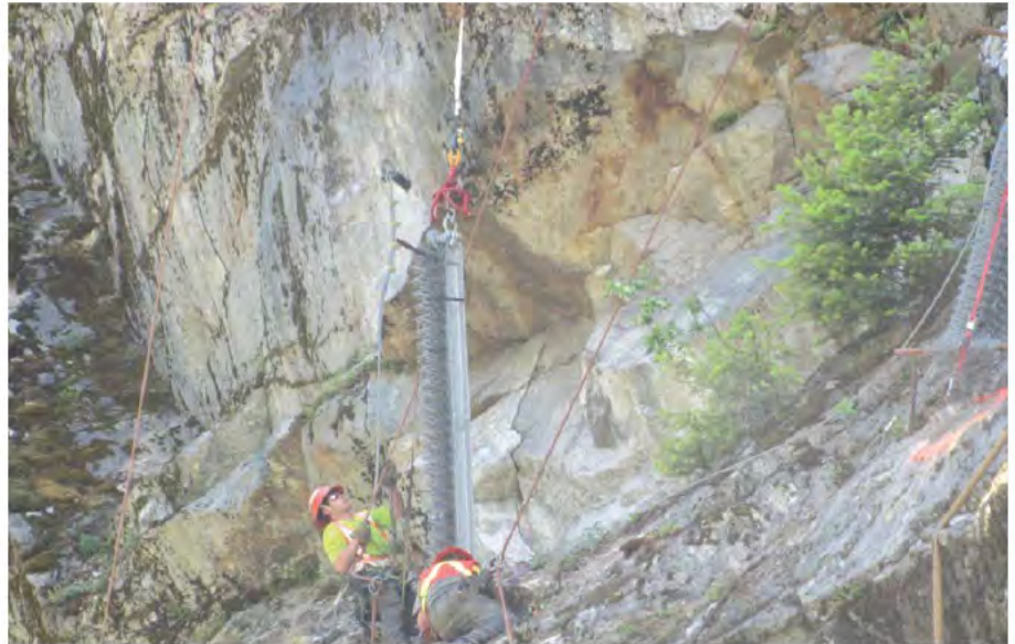
Installation of the rockfall barrier post positioned by helicopter
