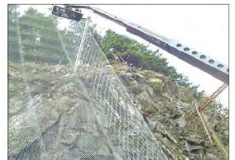
Top: 20 m manlift crane in action for the installation
