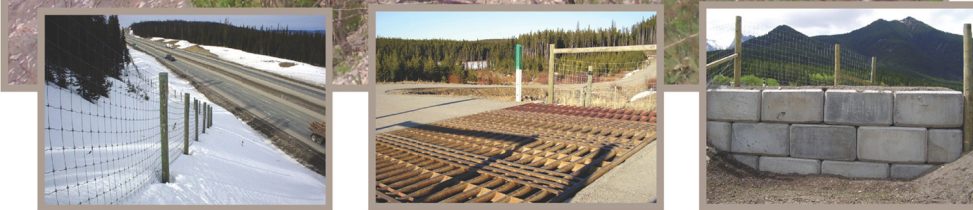
Bighorn sheep and other animals are commonly found near the highway. Extensive exclusion fencing (left), combined with ungulate guards (centre) and one-way escapes (right) will greatly reduce wildlife collisions.
