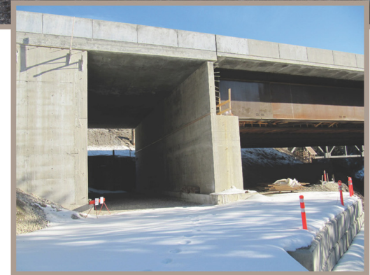
RIGHT: At the new Mount Hunter Creek Bridge, passage is also provided under the highway, under both the long span across the river and the short span between the riverbank and the bridge abutment.
