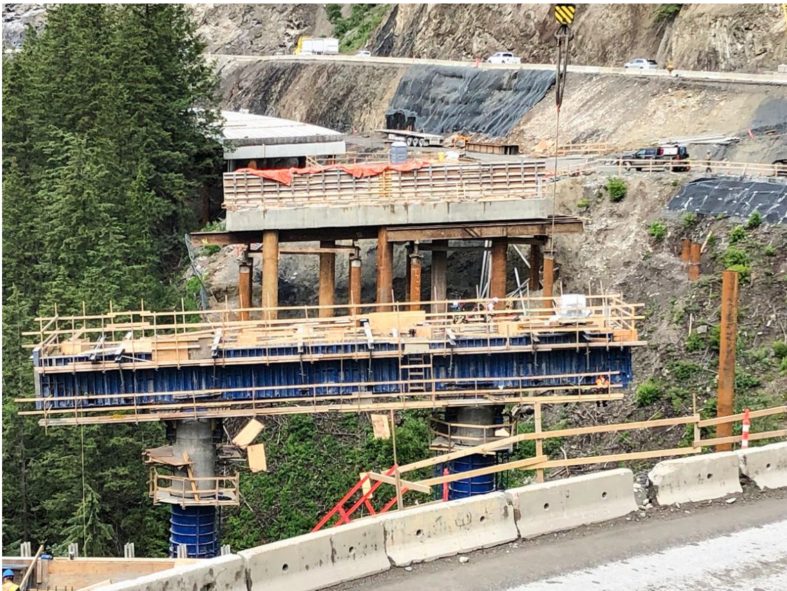
Blackwall Bridge June 2022: Formwork being removed from pier caps
