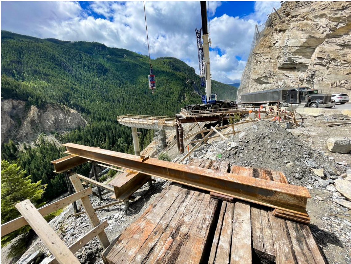
Frenchman's Bridge June 2022: Apparatus being prepared to install girders
