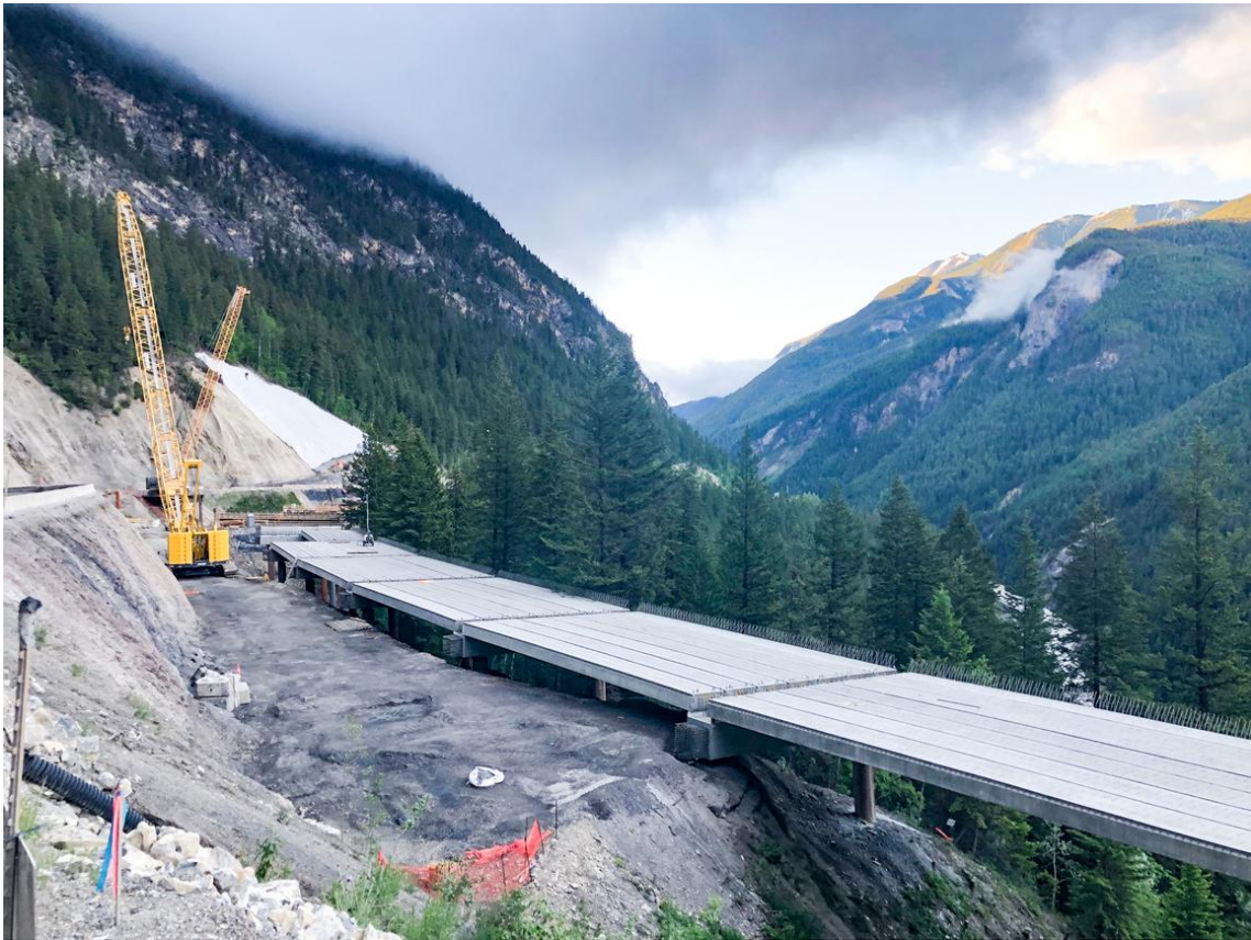
Grizzly Viaduct June 2022: Concrete girders being installed
