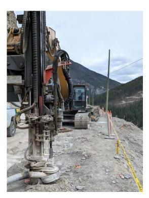
Steep, unstable slopes descending into the canyon require stabilization with soil nails before heavy equipment can move in to
